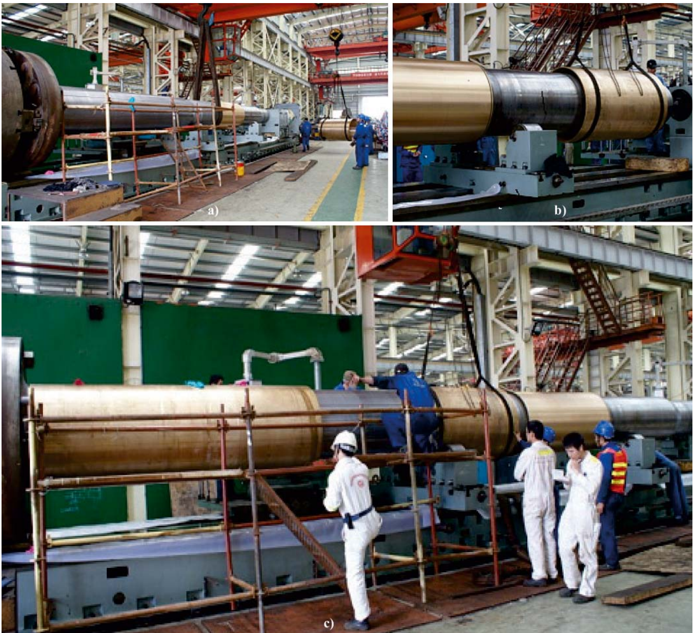
Fig. 6. Run of putting the particular sections of the bearing sleeve onto the shaft
