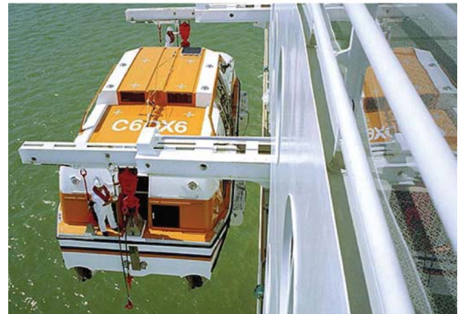
Fig. 5. Photos of the life boat davit fitted with a telescopic mechanism for putting the boats overboard. Left - in voyage position; right - in overboard position.
