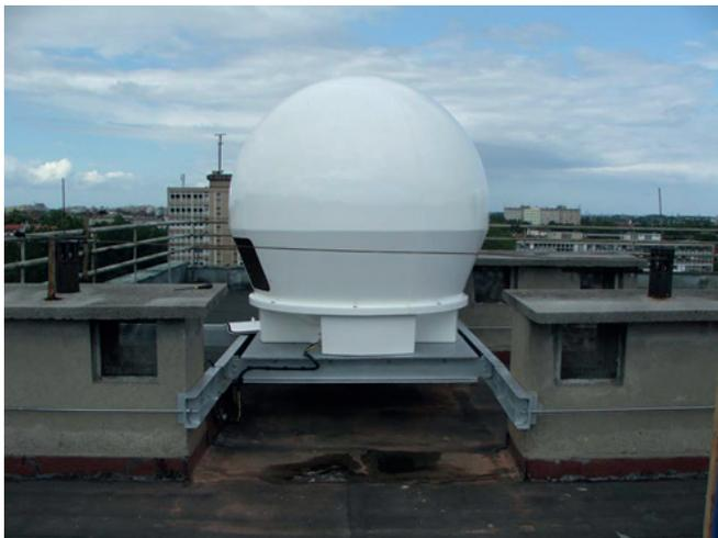
Fig. 1a. 1.5 metre HRPT-MetOp antenna in radome
