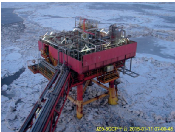
Fig. 2. Typical jacket platform in Bohai Bay
