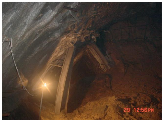
Fig. 5. Intrusion of surrounding rock and primary support in clearance limit of subsea tunnel
