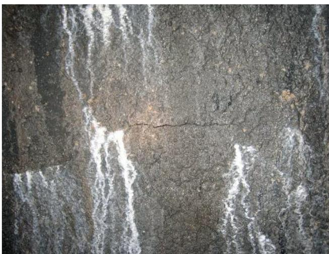
(b) Cracking and water seepage of primary support
