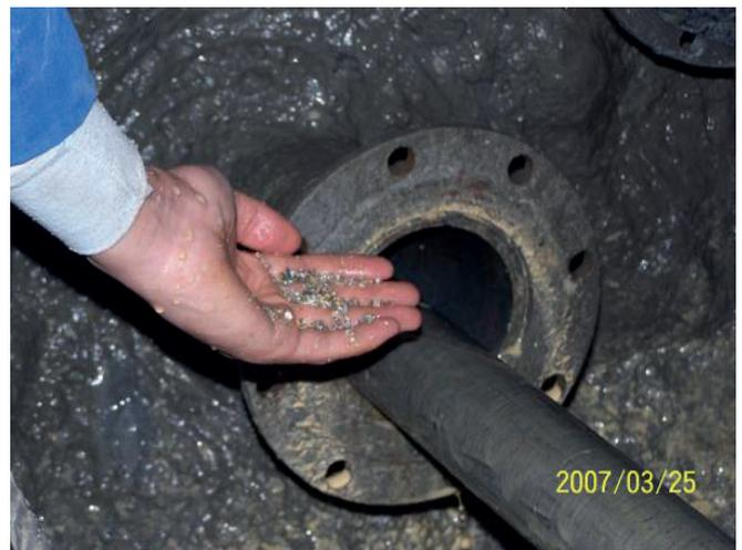
(b) Tunnel water disappeared after grouting
