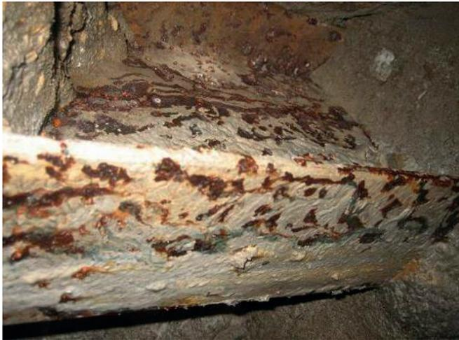
Fig. 8. Steel corrosion in primary support of subsea tunnel
