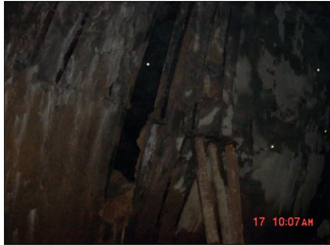
Fig. 4. Concrete peeling and steel arch distortion of primary support in subsea tunnels
