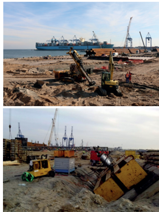
Fig. 6. Production of micro-piles (upper photo), load tests (bottom photo)
