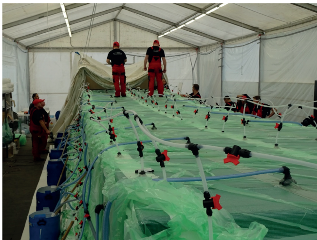
Fig. 2. Preparation to infusion of a large-size object - footbridge span of Fobridge grant
