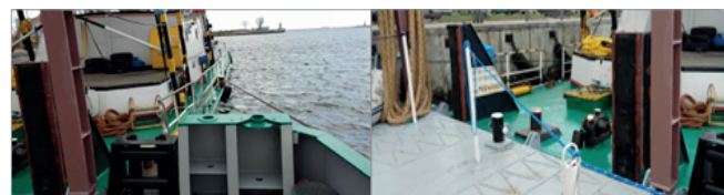
Fig. 1. Push barge – pusher boat “Hetman” and barge “Galar-2” coupling system including cable lines and hydraulic cylinders, on the Lower Vistula River in April 2017
