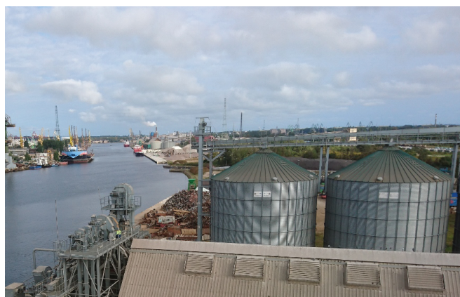
Fig. 1. Battery of steel silos in the Port of Gdansk
