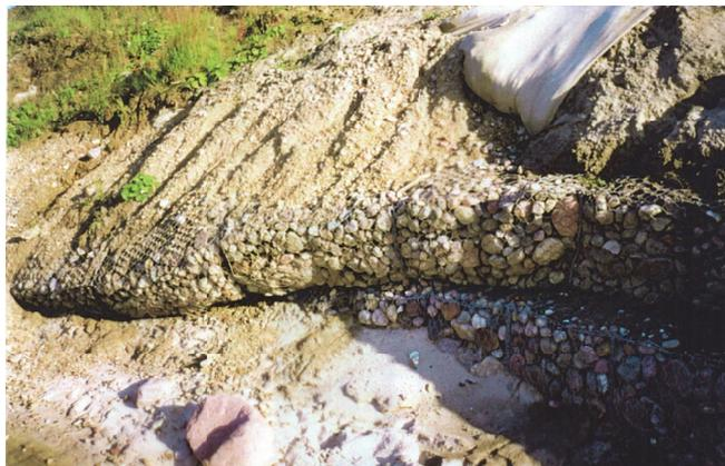
Fig. 3. Gabions composing the seawall in the region of "Bałtyk", damaged in 1998
