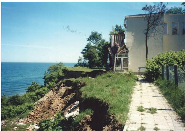
Fig. 2. The leisure centre "Horyzont" situated on the edge of an active cliff and damaged in 2002.
