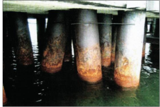
Fig. 6. Sea corrosion of piles [10]
