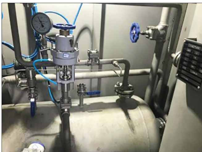
Fig. 2(a). Spiral-wound heat exchanger
