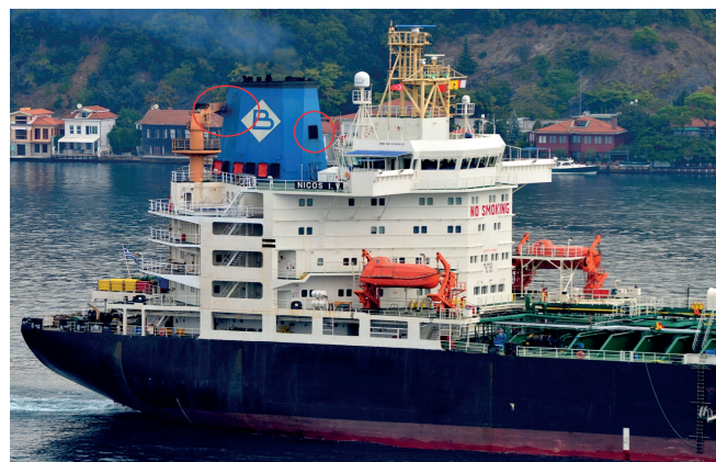
Fig. 10. Superstructure of a tanker with a deadweight of 45,564 t with inlet louvres
