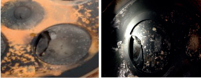
Fig. 3. View of a defective inlet valve of the Deutz 68M628 main power engine.
