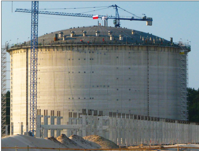
Fig. 1. View of the tank during its construction
