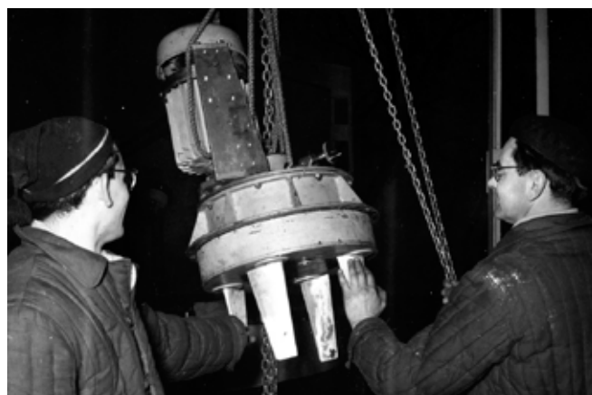
Phot.2 Cycloidal propeller before installing on a tug model
