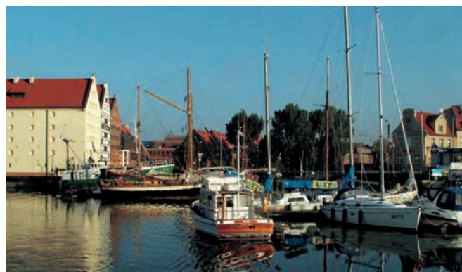
Fig. 5. Gdansk marina in Szafarnia street (own photo, August 2006).
