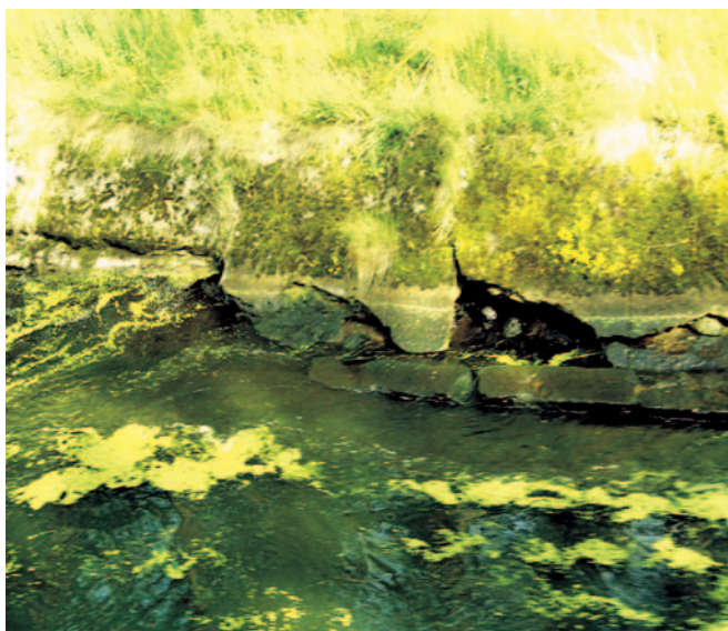
Fig. 1. Difference of water level on canal slope due to ship motion .
