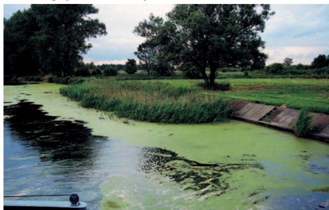
Photo 6. (J. Kulczyk, R. Werszko) The overgrown outer harbour of Sluice no. 4 at Frydrychowo upon the Upper Noteć Canal .
