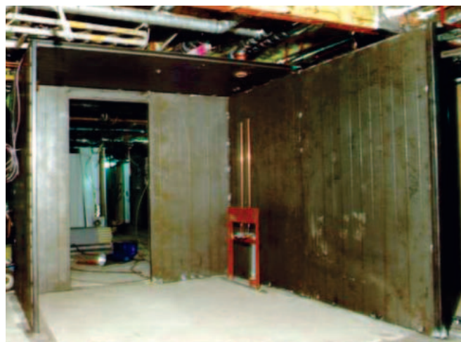
Fig. 2. Internal superstructure walls made of steel sandwich panels (source: Internet)
