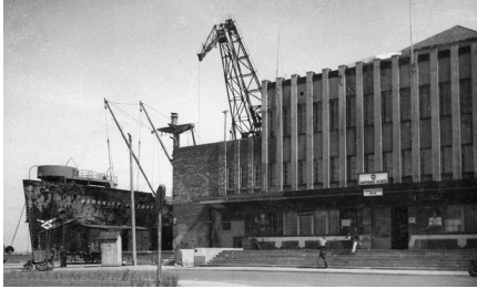
Fig. 3. Gdynia, 1 Polska Street, Maritime Station in 1946. The damage visible in the north-western corner of the building was caused by the Allied air raid of 1943 and was repaired only in 2013–2015, during the comprehensive conversion of the building into the Emigration Museum. After the war, until 1963, the Harbour Master's Office was located in the Maritime Station; source: Gdynia City Museum; photo: Jan Bułhak.
