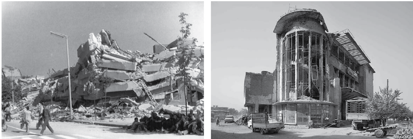
Fig. 3. Destructions of the Skopje earthquake 1963 (source: Skopje1963_ plostad-sloboda@public domain). Fig. 4. Destroyed cinema in Kabul, Afghanistan, c. 2012 (source: Jean Molitor_highres, 2012).
