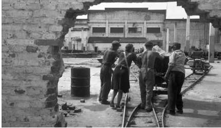
Fig. 2. Gdynia, demolition of the damaged Cukroport III/IV warehouse at the Polish Quay in 1946. Through the large breach visible in the warehouse wall, the façade of the Cukroport I/II warehouse can be seen. The works were carried out using temporary rails; source: State Archive in Gdańsk, Gdynia Branch.
