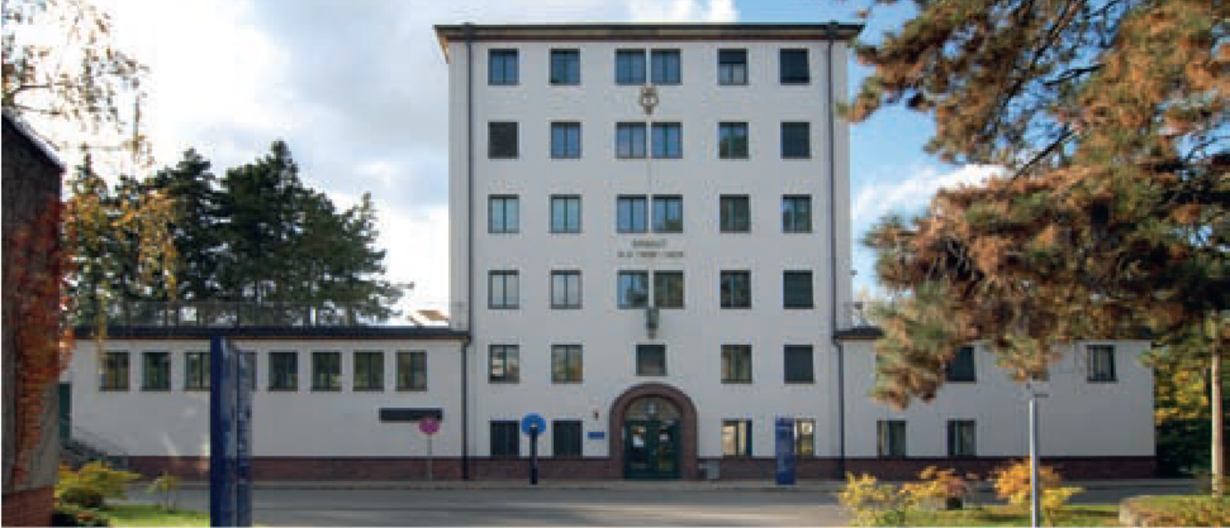
Fig. 11. Entrance tower block to the campus of the Kaiser Wilhelm Institute for Brain Research in Berlin–Buch, built 1928–1929 according to plans by Carl Sattler, the institute building on the outskirts of the city was occupied in 1931 (source: Landesdenkmalamt Berlin, photo Wolfgang Bittner).
