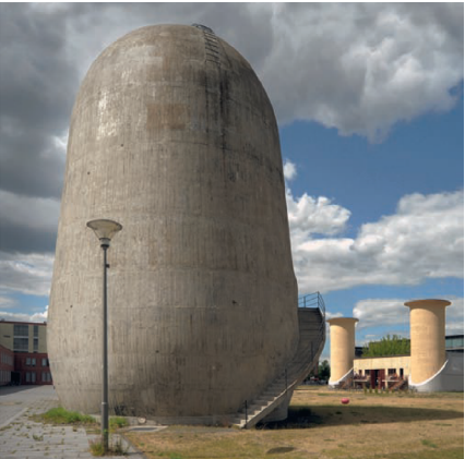
Fig. 12. Reinforced concrete shell buildings of the aerodynamic test facilities of the German Aerospace Research Centre (DLV) in Berlin–Treptow (Johannisthal/Adlershof), built in 1932–1940, designed by Hermann Brenner (1899–1969) with Werner Deutschmann (source: Landesdenkmalamt Berlin, photo W. Bittner 2010).
