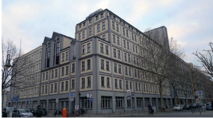
Fig. 15. The expressionist corner building of the headquarter of the General German Trade Union Federation (ADGB) in Berlin–Mitte ( Wallstraße/Inselstraße ), by Max Taut and Franz Hoffmann (1922–1923) (source: photo Shaun92, https://commons.wikimedia.org/wiki/File:Adgb-gebaeude01.jpg?uselang=de%20(2021)BB_Bundesschule_der_ADGB_Bild1_ADBG_e88c8fbf5e.jpg ).
