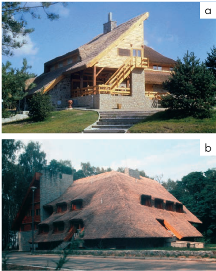
Fig. 8. Examples of inns/motels built according to the design of architects J. Buszkiewicz and J. Kopydłowski from the mid–1970s: a) inn–motel located on the national road E8 (source: Herder–Institut Marburg, Bildarchiv, Sammlung Orth, Nr. 209387); b) Wielkopolska inn located by the E8 road, 1974 (source: Herder–Institut Marburg, Bildarchiv, Sammlung Orth, Nr. 208426).
