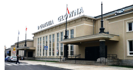
Fig. 9. Gdynia, the new railway station, construction 1950, arch. Waław Tomaszewski, (photo Maria Jolanta Sołtysik 2012).
