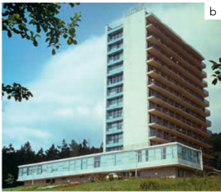
Fig. 11. Examples of Polish sanatorium designer in the 1960s: a) Ustroń-Zawodzie, sanatorium complex, 1967–1990, Dom Lecznico-Wypoczynkowy 'Narcyz' (source: KAW postcard, photo by J.Malinowski); b) Szczawnica, sanatorium 'Hutnik', 1963 (source: Herder-Institut Marburg, Bildarchiv, Sammlung Orth, Nr. 208517).
