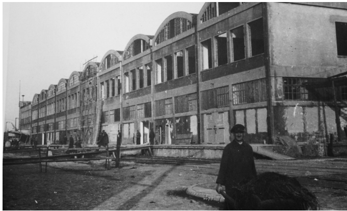
Fig. 4. Gdynia, 1 Polska Street, southern façade of the Maritime Station in 1945: a) visible alterations to the original layout in the form of window openings made by the Germans during the occupation; b) visible row of windows bricked up during renovation, with blinds left in place; these were removed in 2015 during the conversion of the building into the Emigration Museum; source: State Archive in Gdańsk, Gdynia Branch; photo: W. Glasko.
