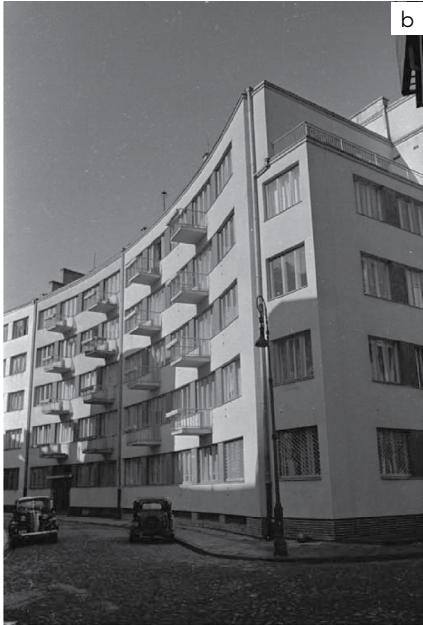
Fig. 12. a–b) Stockholm, Sweden, Congress of the International Federation for Housing and Urban Planning (IFHTP), July 1939. Unidentified apartment building in Visby [?]; photo: S. Syrkus; source: ZAP WAPW collection.
