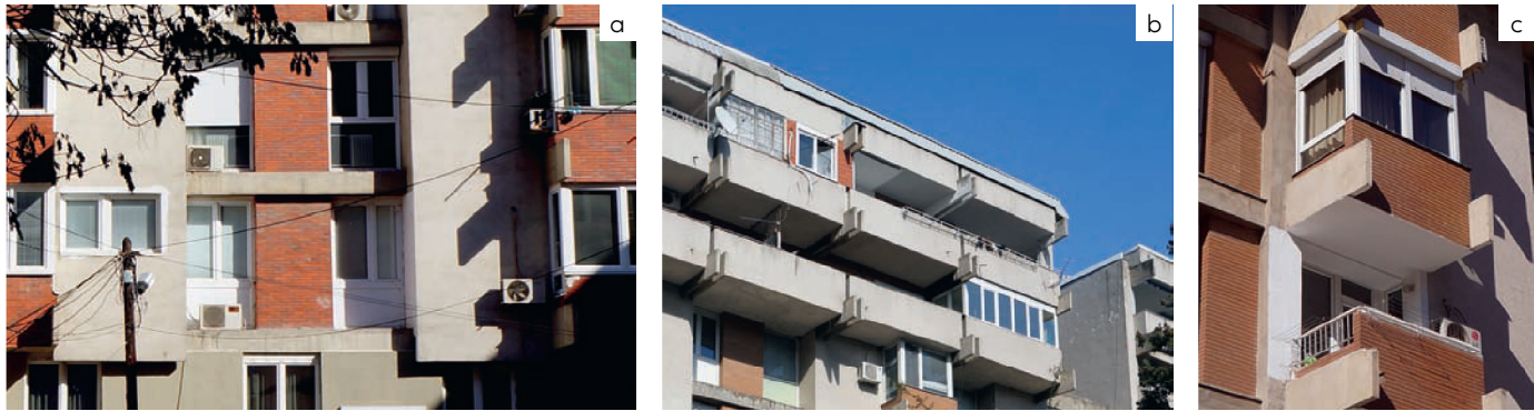
Fig. 7. a–c. Alterations carried out by the dwellers, including sloped roof cover, enclosing parts of the terraces, adding new balconies, turning bay windows into balconies and other changes and additions to the facades. © Vlatko P. Korobar, 2023.
