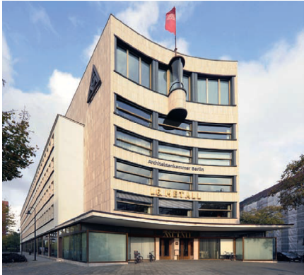
Fig. 16. German Metalworkers’ Trade Union Centre (DMV Haus) in Berlin–Kreuzberg (Hallesches Tor), built in 1929–1930, arch. Erich Mendelsohn and Rudolf Reichel: the glazed meeting room on the top floor has a speakers pulpit, which is orientated towards both the interior of the building and the space in front of it (source: Landesdenkmalamt Berlin, photo W. Bittner 2015).
