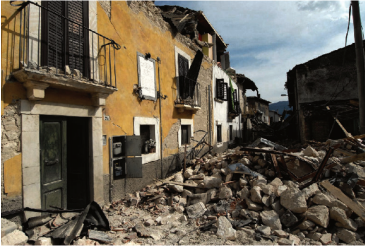
Figure 1. Structural Damage during the Mw 6.3 Abruzzo Earthquake in 2009
