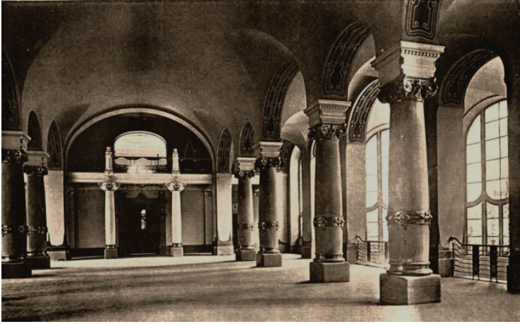
Figure 12a. Upper Hall with the entrance to the Lecture Theatre
