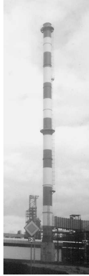
Figure 2. Overall view of the chimney
