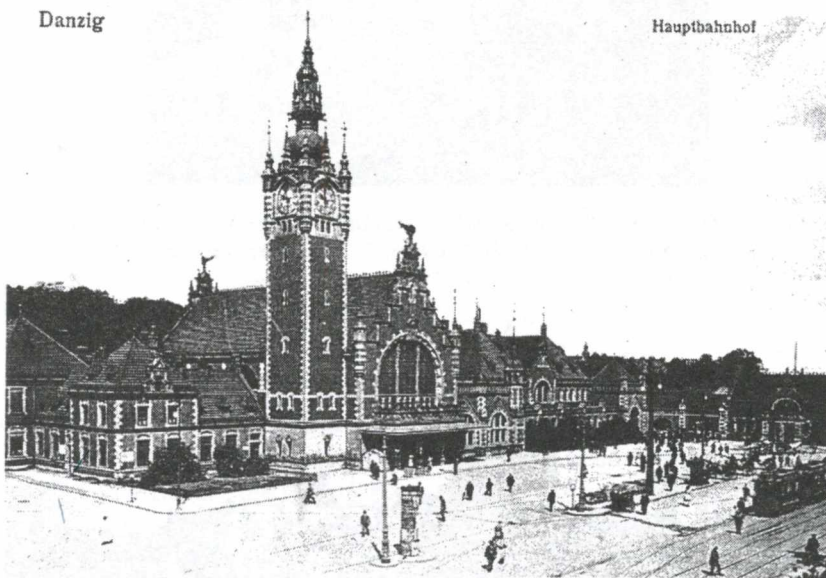
Figure 9. The Main Station in 1900. We can see the beautiful shapes of the roofs in the side wing — not rebuilt until now
