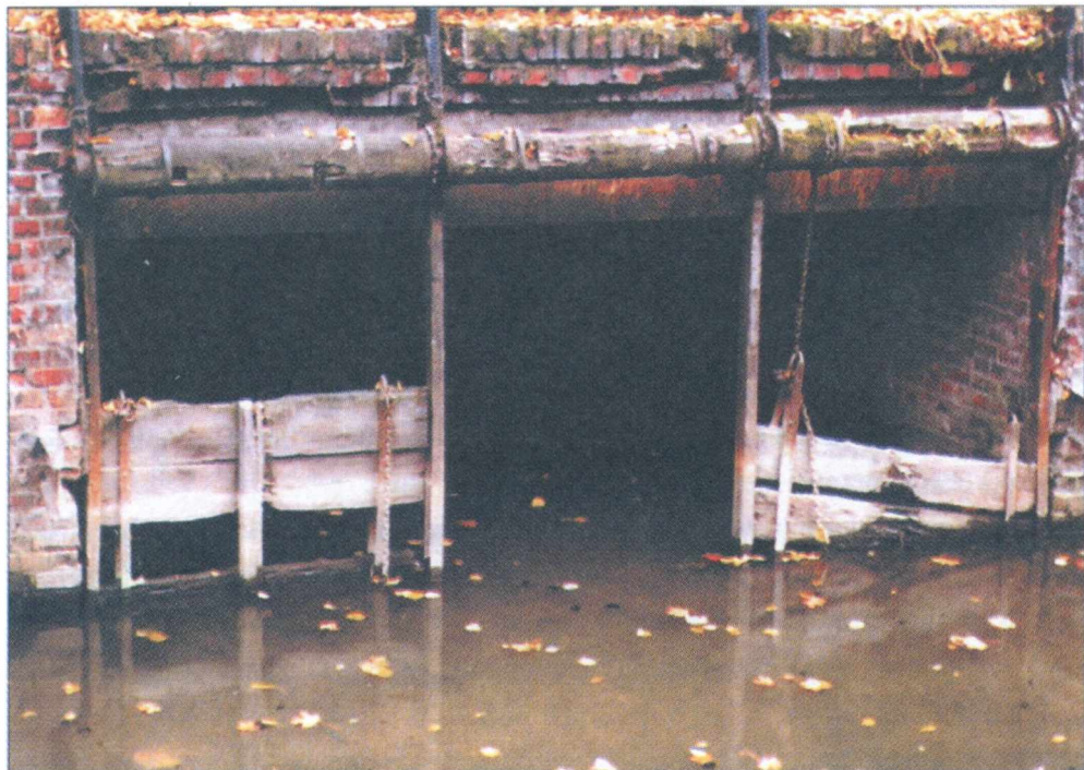
Figure 8. The sluice gate letting water into the Small Mill Canal on Piaski — the present state
