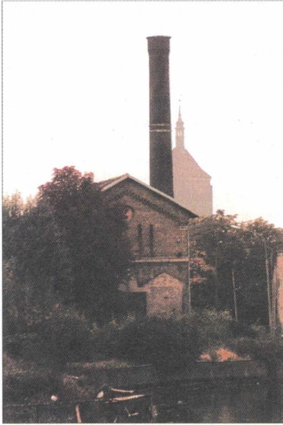
Figure 15. The historical sewage pumping station on Kępa — the present state
