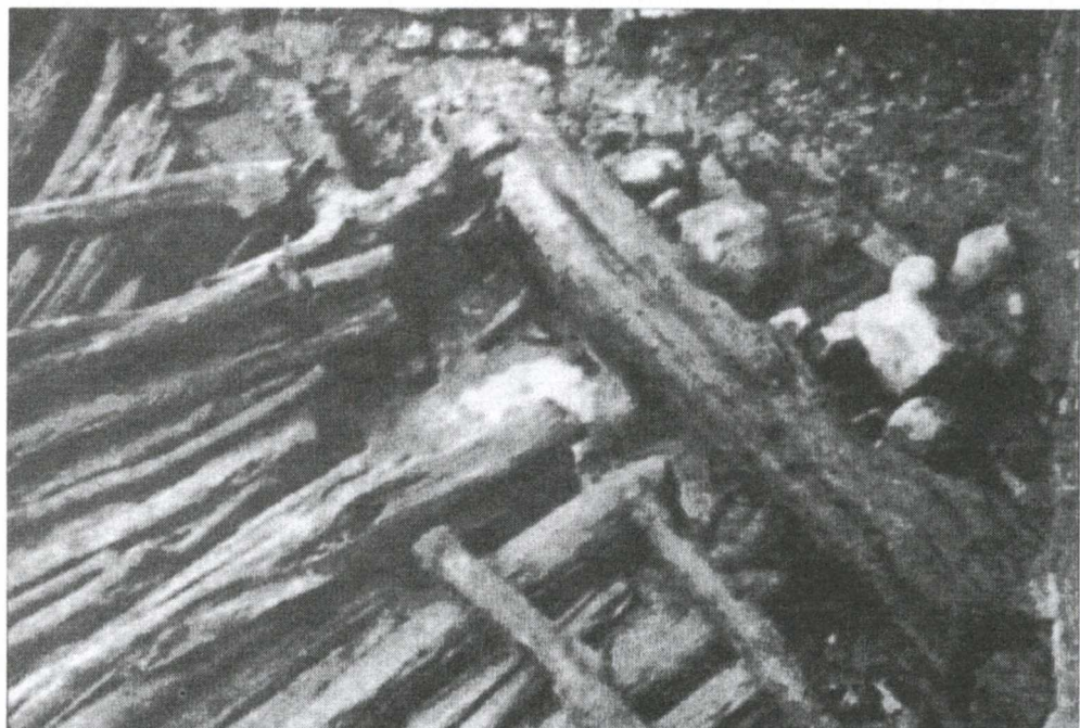
Figure 9. Construction of the oldest quays.
