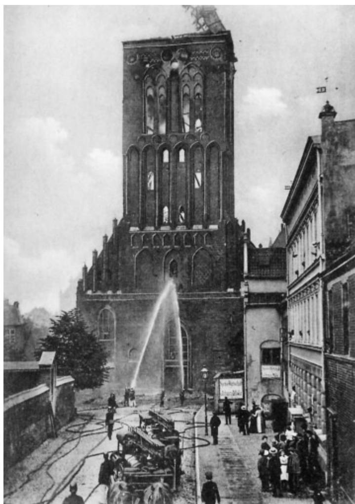
Figure 1. Fire at St. Catherine's Church in 1905
