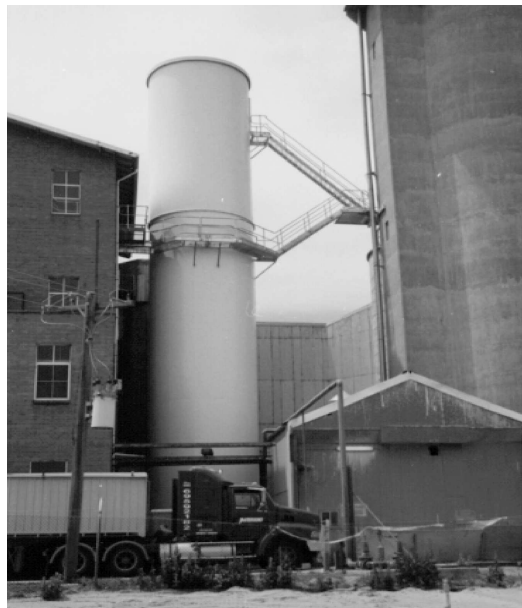
Figure 12. 200 tonne wheat conditioning silo
