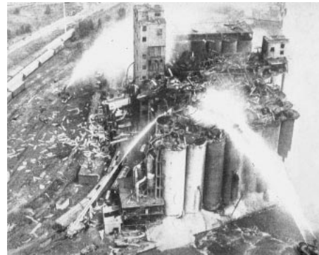
Figure 3. Rolands-mill Bremen after dust explosion
