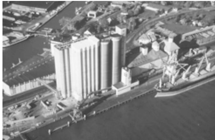
Figure 14. Overview of the plant
