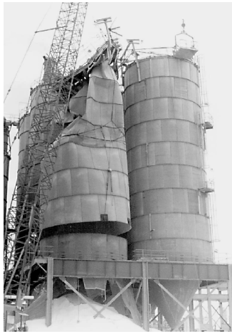
Figure 9. When mass flow develops in a funnel flow silo, the results can be catastrophic
