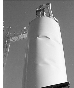
Figure 3. Silo deformation
