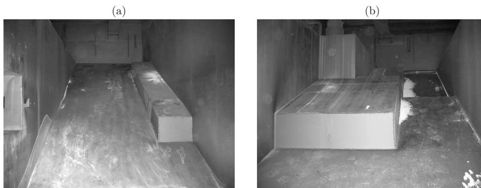
**Figure 2.** Photographs of the inlet space of (a) the side windbox and (b) the middle windbox with obstacles installed in the way of the air stream
